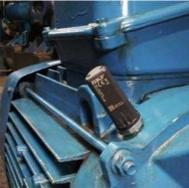
SKF Enlight Collect IMx-1 is a scalable and easy to set up mesh sensor network for data collection, available on a fee-based contract
